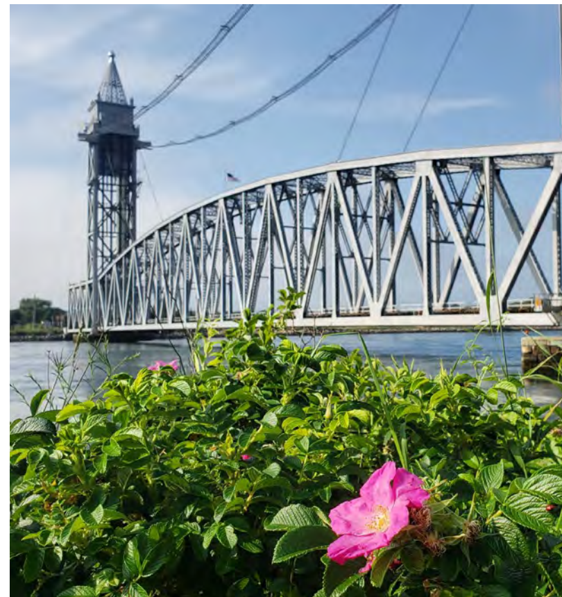
Cape Cod Canal Railroad Bridge, Bourne
