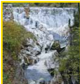
Marble Dam at Natural Bridge NORTH ADAMS
