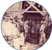
Tunnel workers ready to descend the Central Shaft
